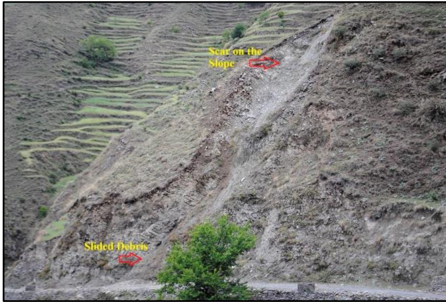
Photo plates (1 and 2): Landslides in the Study Area (Source: Field Survey, 2018)
